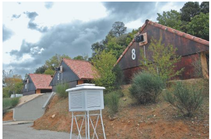
Example of Actis "in-situ" test cells, Limoux, France.
