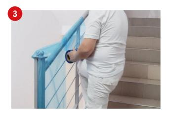
FOLI PROTECT is fully self-adhesive and available in widths of 25/50/100 cm.
